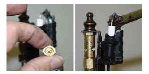
Reverse the procedure to reassemble the pilot burner using pipe thread to avoid gas leakage. Tighten all connections securely.
